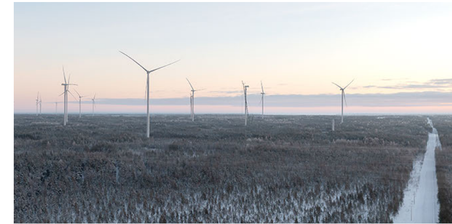
Metsälamminkangas Windfarm (2) ~200 GWh p.a. net power generation
